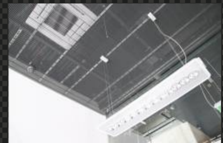
Air-conditioning and ventilation
