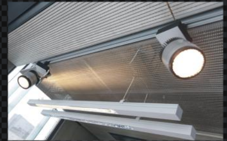
Lighting and sound system
