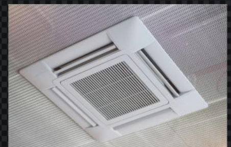
Air-conditioning and ventilation
