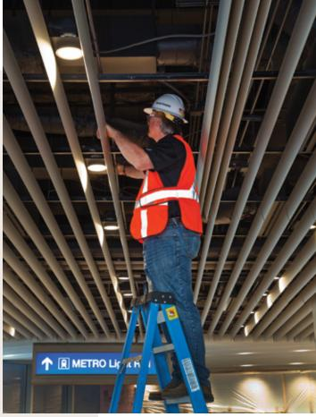
The High Profile Series creates a clean plenum mask that offers easy point access to lighting, HVAC, security, audio and fire safety systems. Baffles easily slide or demount to allow hassle free access for maintenance. The spacious appearance is ideal for large interior spaces, when a more open ceiling plane is desired.
